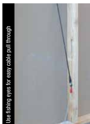
Drill vertically through noggins and plates
