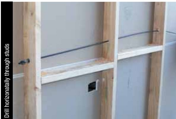
SuperFlex positioning handle for accurate drill positioning
