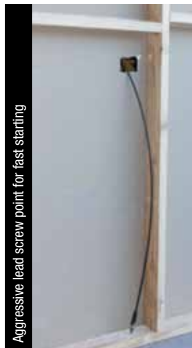
Use fishing eyes to attach cables/wires for easy pull through
