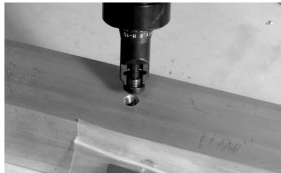
You are now ready to place the nozzle of the tool on the tapped hole and install the insert.
